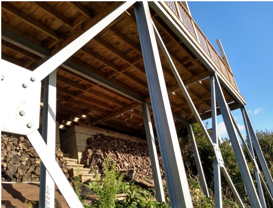
Figure 5: current position of supporting posts
